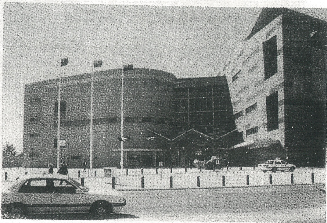
Fig. 7 Main entrance view of Te Papa on completion
