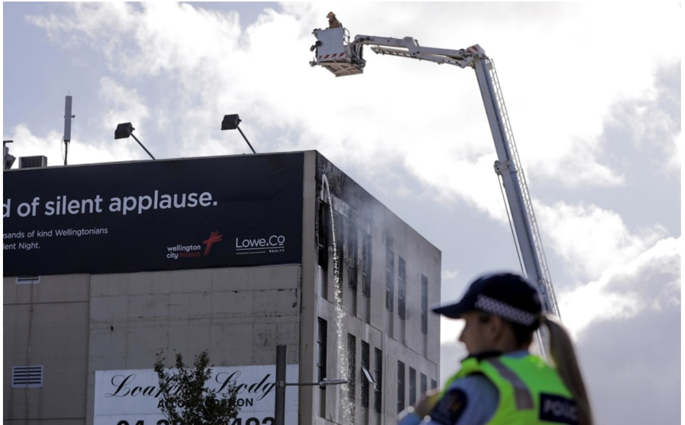
Firefighters at the scene of the Loafers Lodge fire in Newtown. Photo: RNZ / Angus Dreaver
