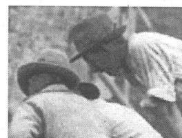
Clearing the rubble
