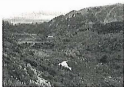
Before: Leader dam 12 December 2016 (looking upstream) (photo: GNS Science)
