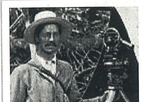
Surveying for the main trunk line
