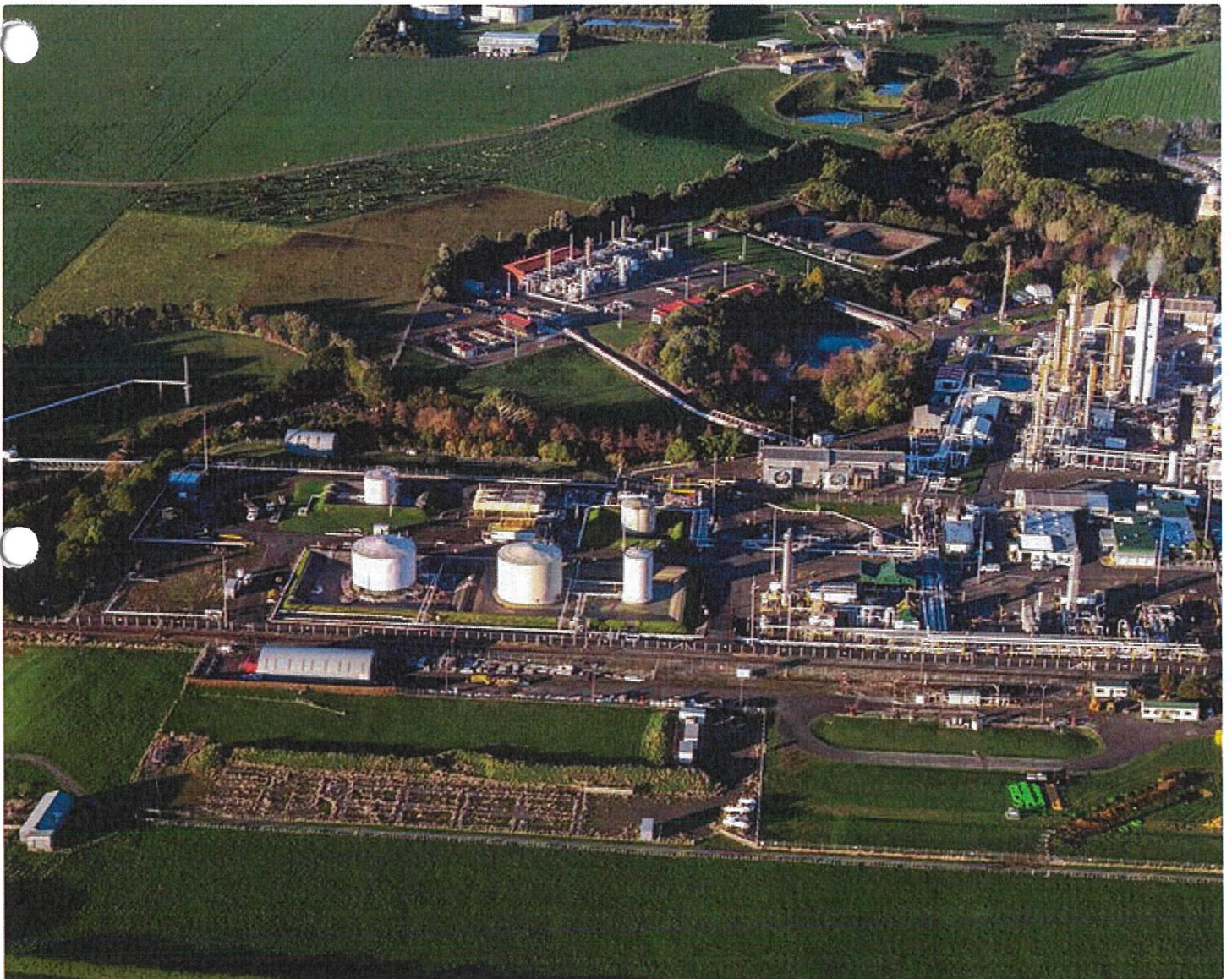
Todd Energy's Kapuni liquid CO2 processing plant. (Source: Supplied)
