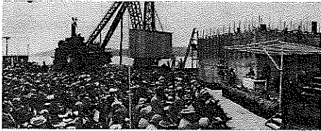
Marking the foundation
